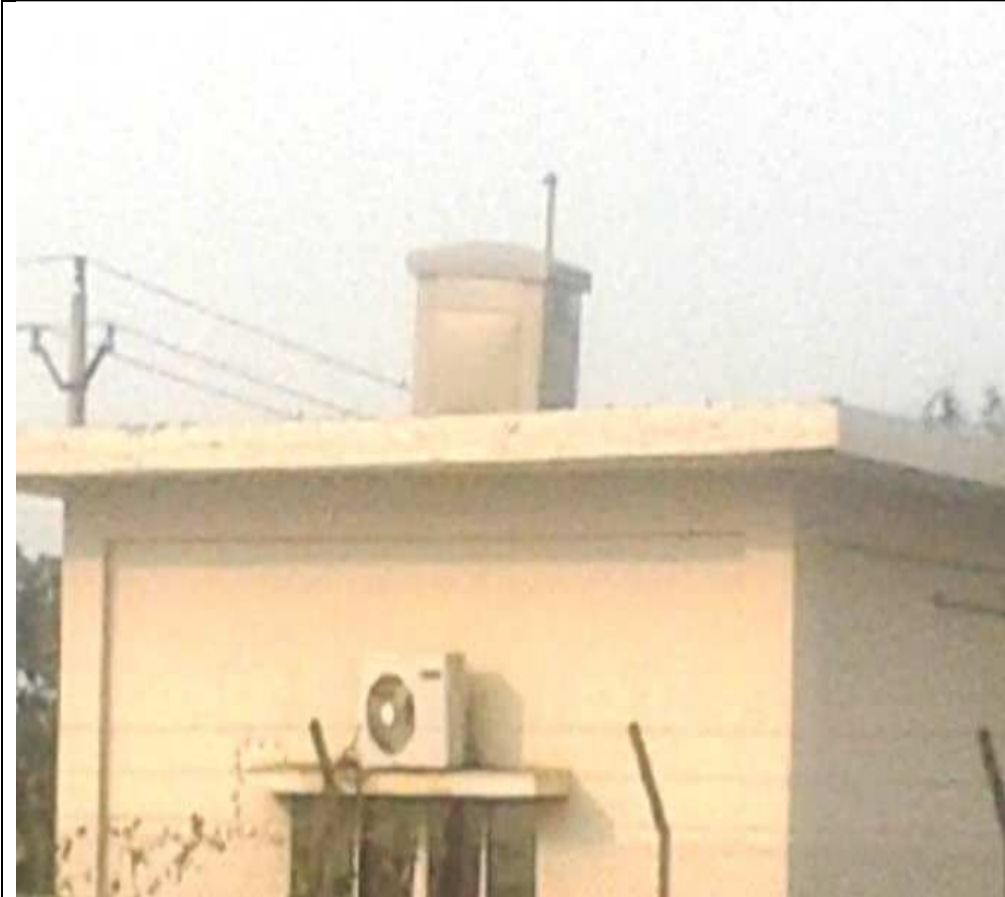
Installed at Sub station
