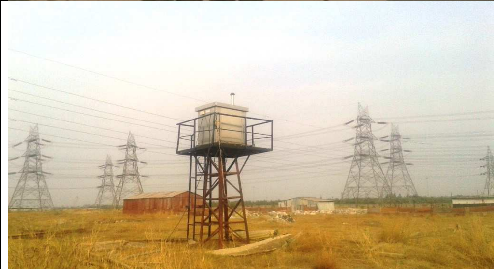
Installed back side to switch yard
