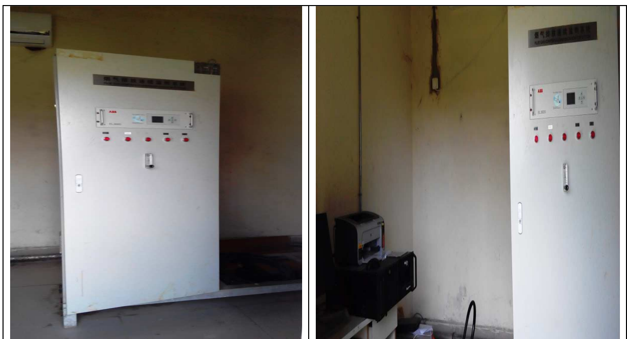
CEMS –II Installed at KSK- MPCL
