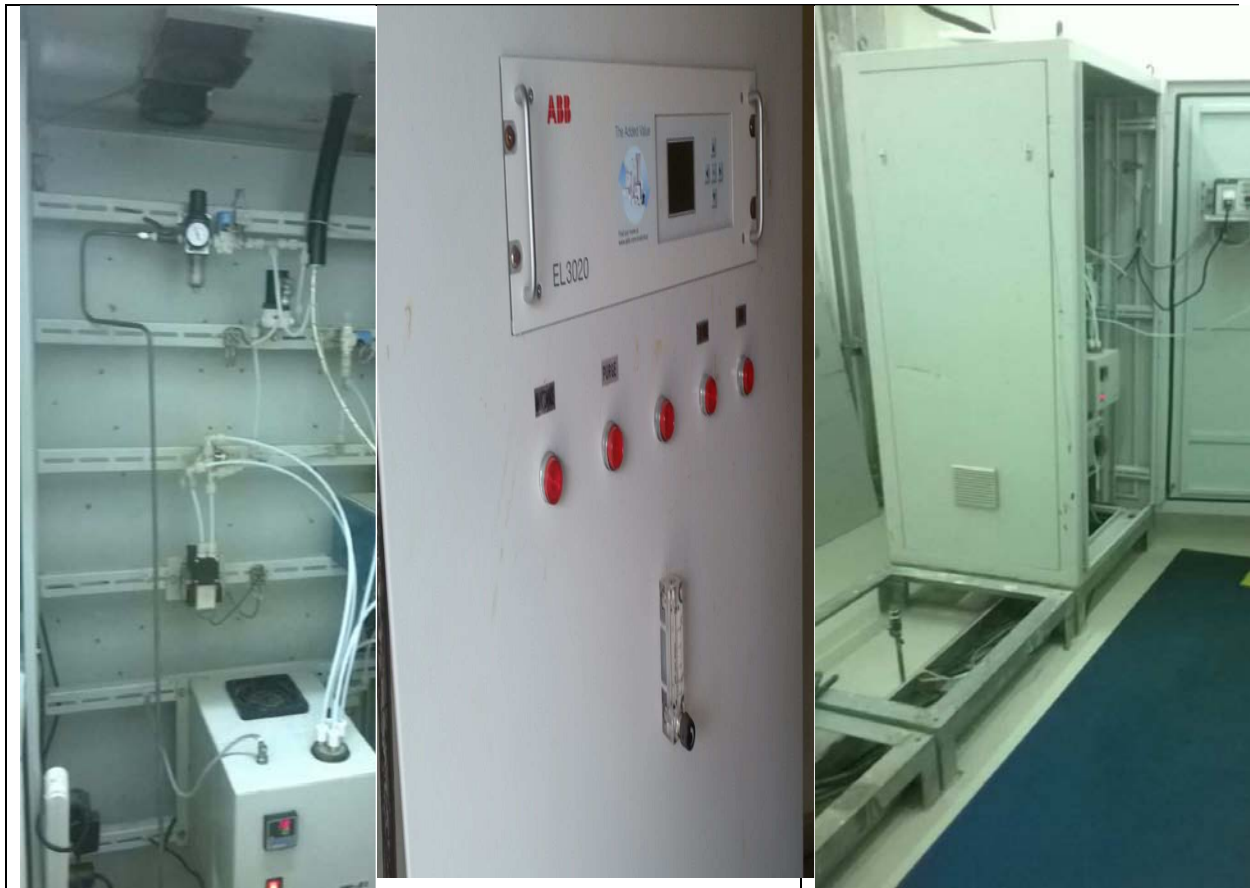
CEMS –I Installed at KSK- MPCL
